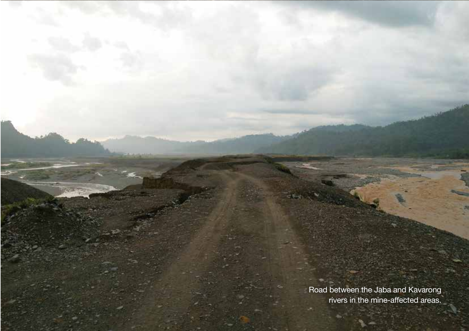
Ruins of the primary crusher from the Panguna mine.
